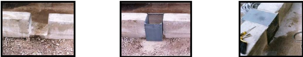
**Figure 6-9: Imbiber Beads® Gravity-Flow Drain Protection System—Curb Application**
